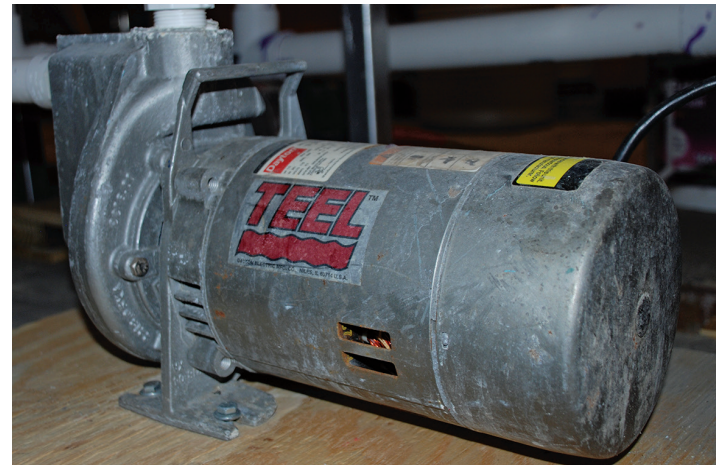
Figure 9. In-line impeller pump.
