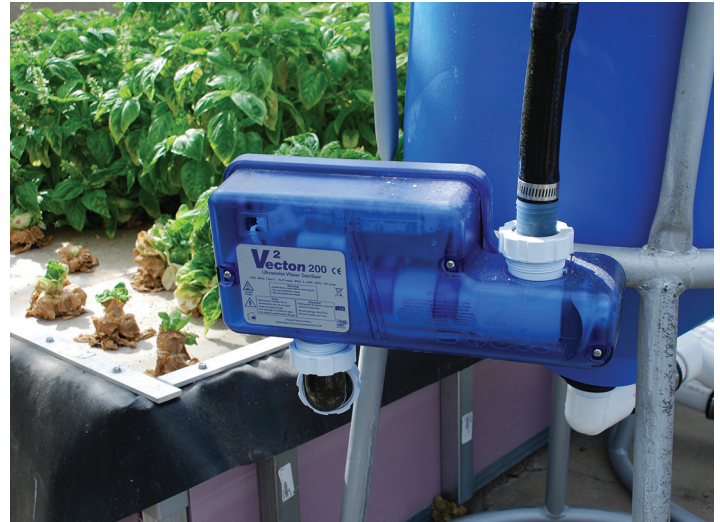
Figure 13. Ultraviolet light sterilizer.
